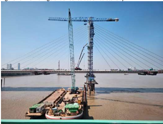
Figure 19: New bridge under construction to StarCity
