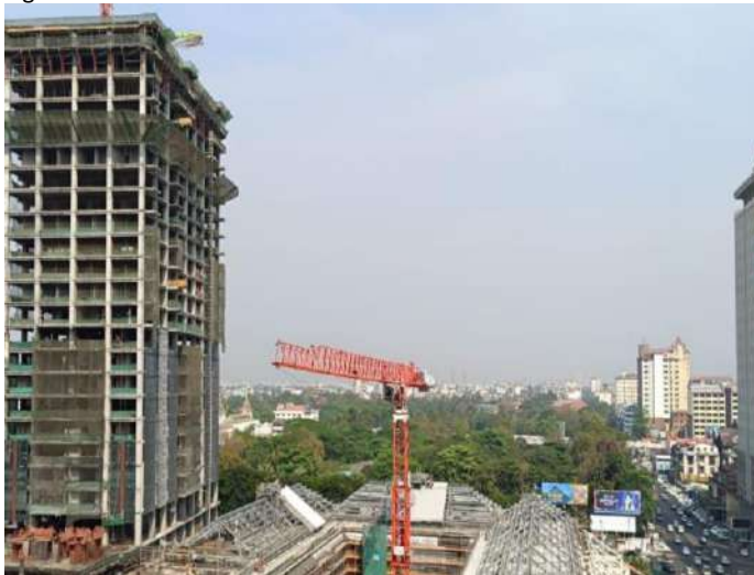
Figure 15: Yoma Central construction site
