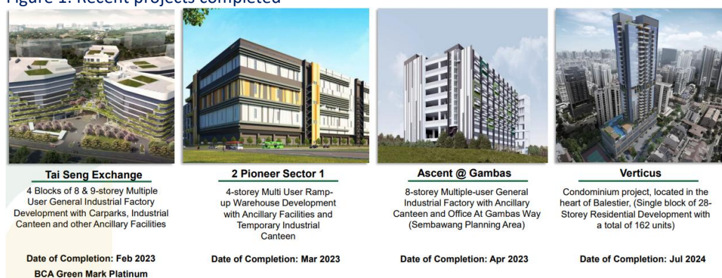
Figure 1: Recent projects completed
