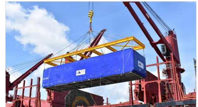
Figure 2: PPVC unit at a construction site
