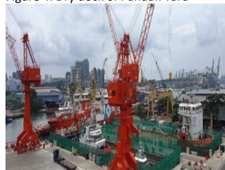
Figure 4: Dry dock of Pandan Yard
