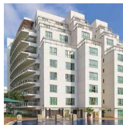
Figure 54: Village Residence Hougang
