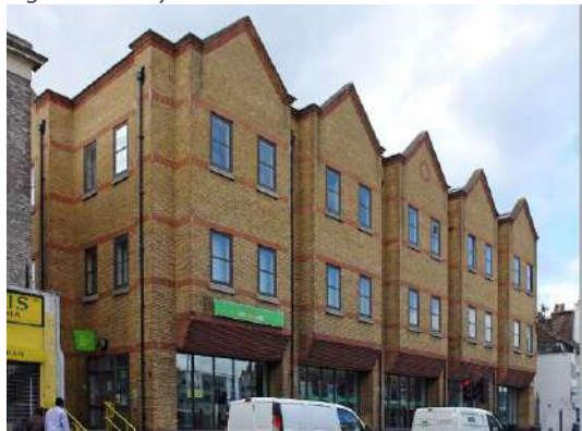
Figure 9: Collyer Court – Job Center
